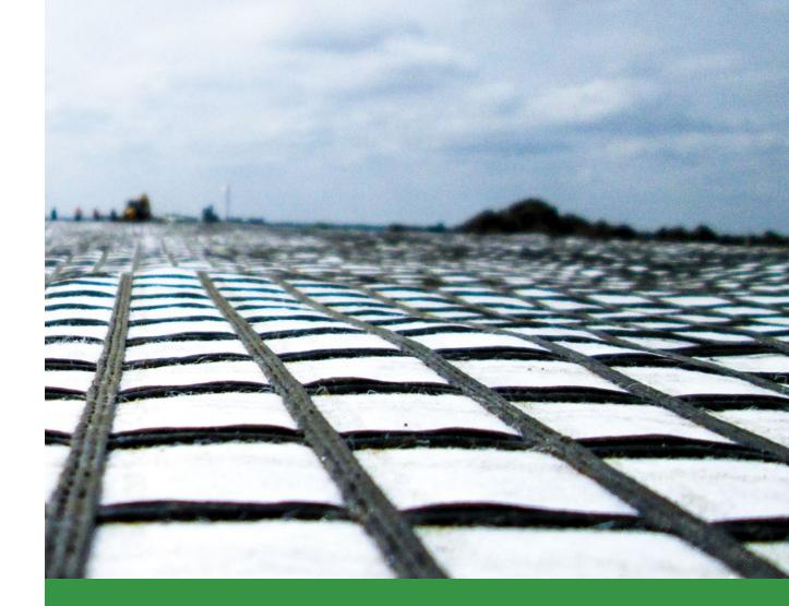
ForTex Geocomposites are developed for bi-axial or uni-axial strength requirements for various applications of civil engineering serves reinforcement, separation and filtration requirements in one product.
